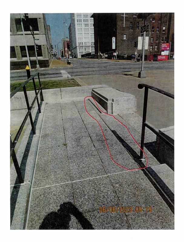
Area circled red is uneven and needs to be leveled to prevent tripping hazard.
