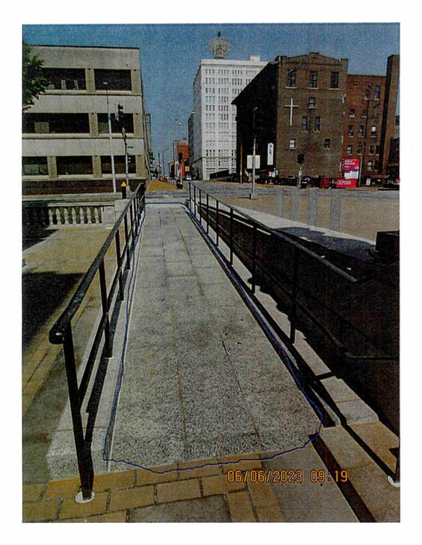
Area circled blue needs missing mortar cleaned and re-tuckpointed.
